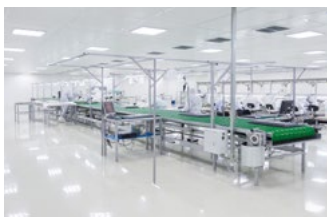
Monitoring and regulation of differential pressure, relative humidity, temperature, air velocity and ACR** in cleanrooms and operating rooms
